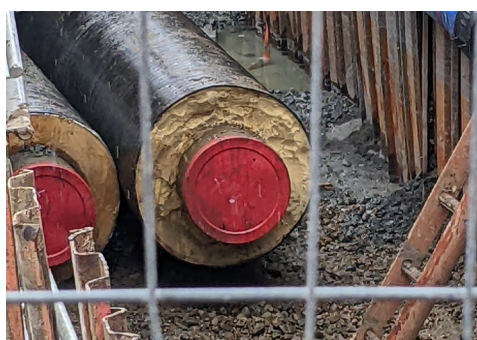
Pipes will carry heated water from the incinerator
